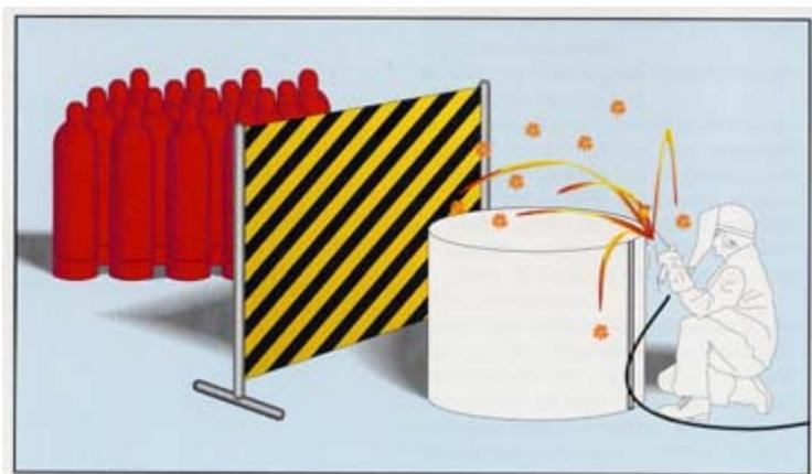
**Figure 4.2:** Example of screening for work giving rise to flying sparks<sup>4</sup>
